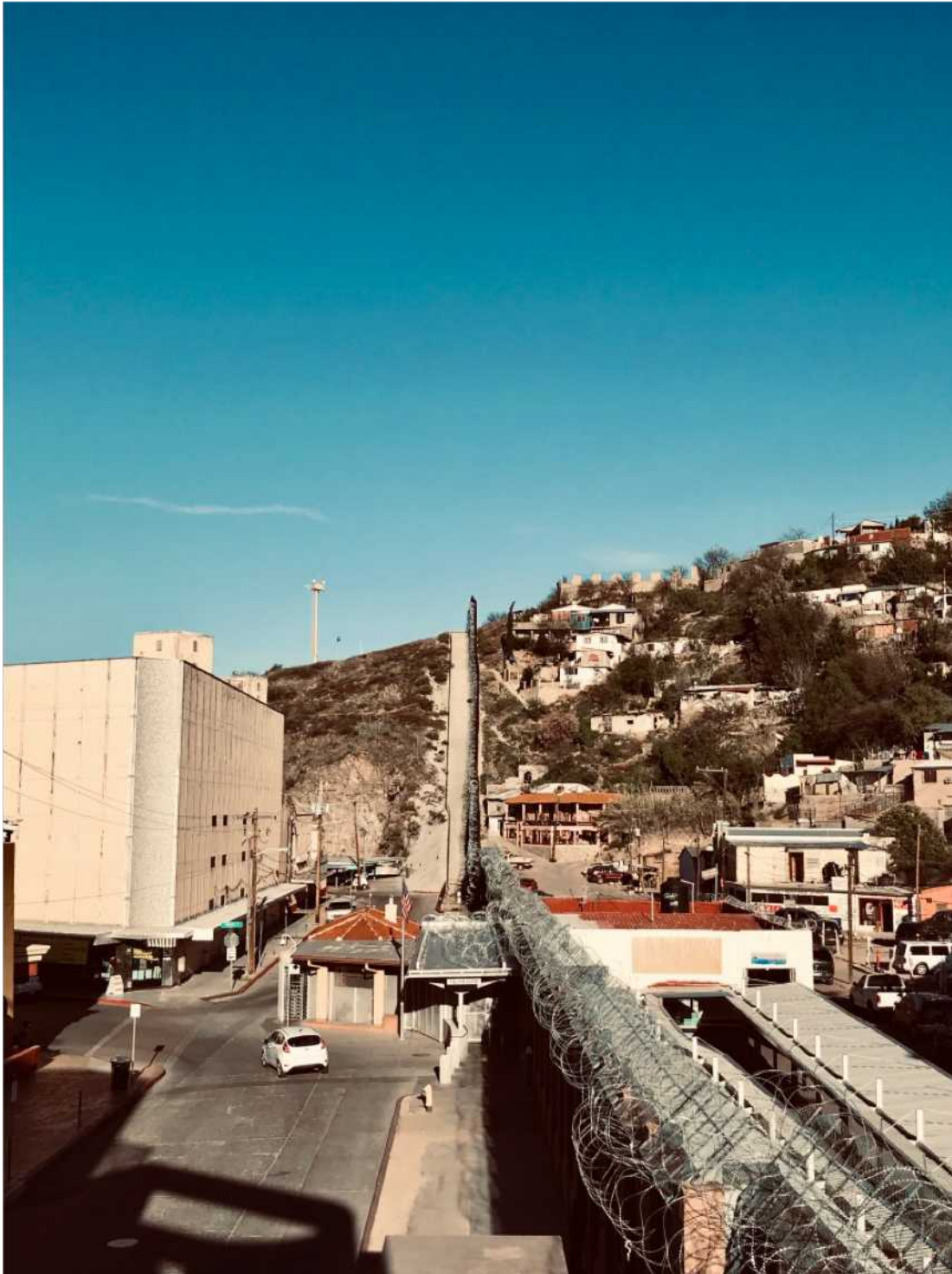
Figure 2: Nogales, Arizona, left, and Nogales, Sonora, right, divided by the US-Mexico border: a concrete and steel fence with newly installed barb wire. Photo: Author, 2019.
