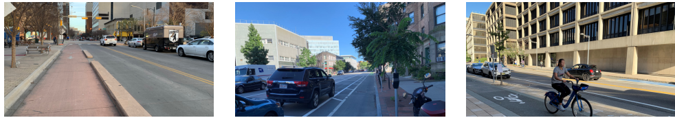
(a) Protected bike lane with a fixed, raised barrier (b) Protected bike lane with parking buffer (c) Raised protected bike lane
